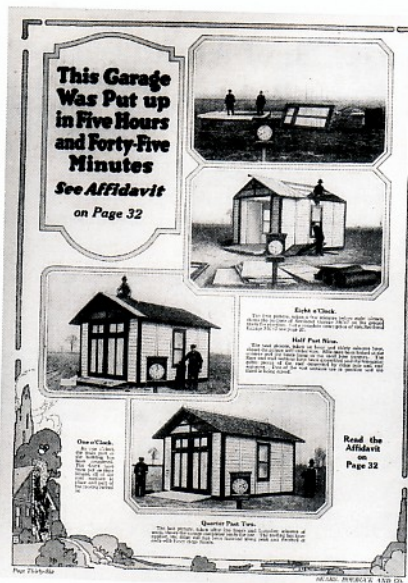
Fig. 5 Advertisement for the Sears Simplex Sectional Garage showing that it could be assembled in less than six hours. Sears offered kits for wood and metal auto houses well into the 1920s.
