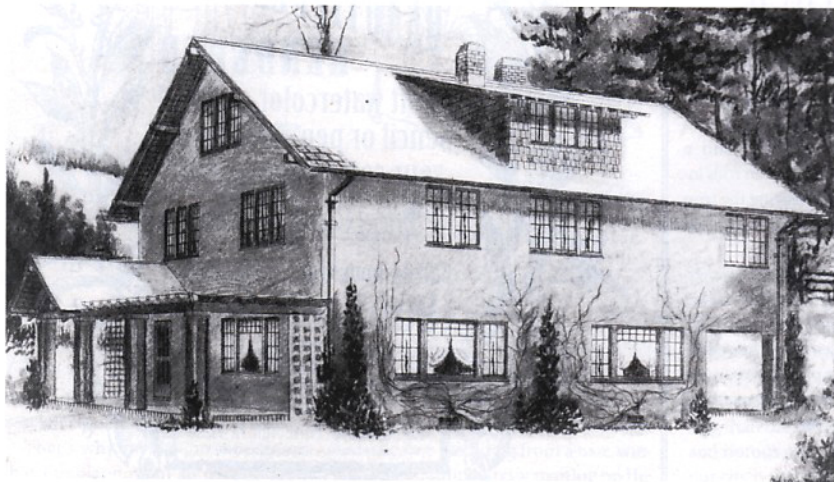
Model No. 154 from the June, 1916 issue of The Craftsman magazine is another gable-front type Craftsman-style home. Its grouped windows and clean surface materials speak of an age of simple, economical yet architecturally satisfying homes. The major bands of windows light the living room and the dining room.
