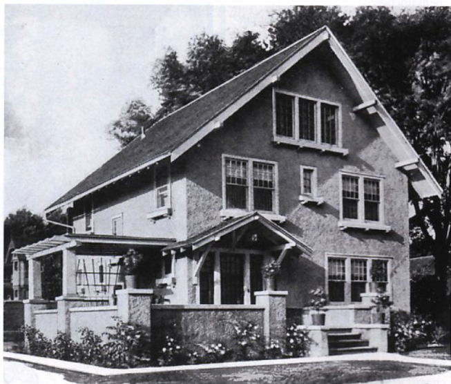
Note the rough stucco finish, side pergola, and stick brackets at the entry in Aladdin Homes' Lamberton model from 1920. Eleven windows and a three-part glass entryway flood the interior with sunlight. The porch is a wrap-around style that combines a covered stoop and a side pergola both connected by a terrace. This four bedroom home was available from 1916 to 1922.
